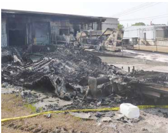
Trailers with organic peroxide products were destroyed by fires at the Arkema facility in Crosby, TX during Hurricane Harvey.
